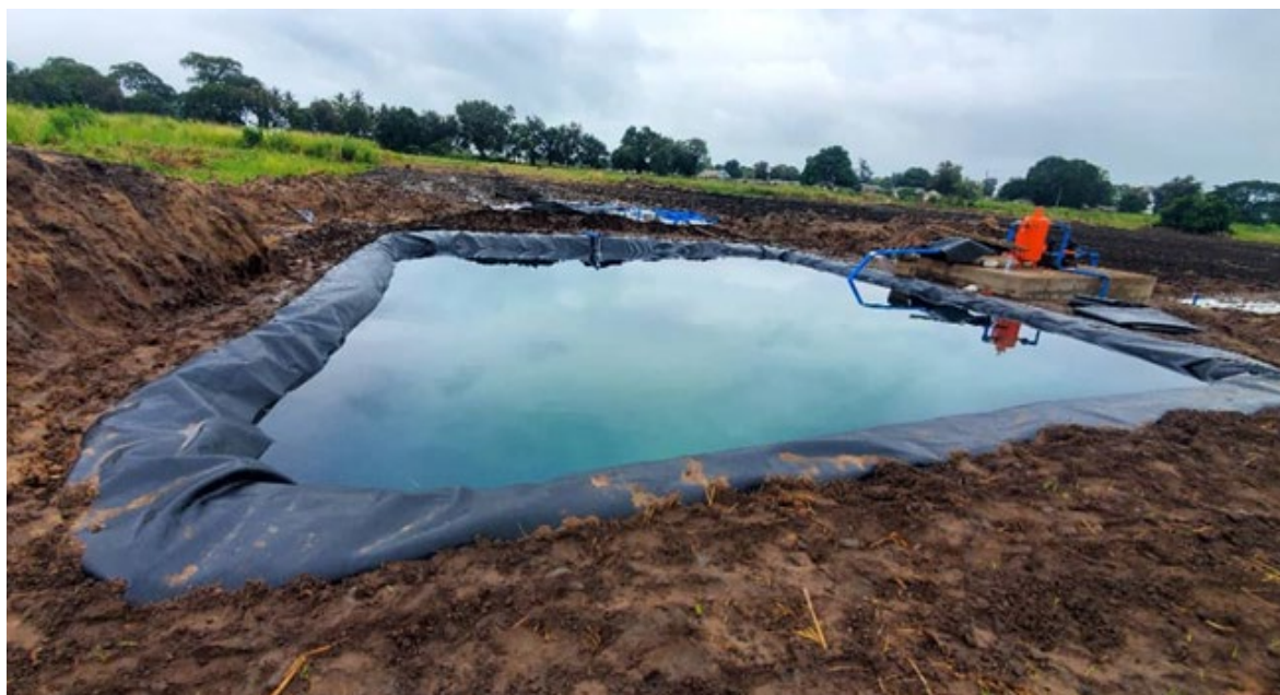
Figure 1: A dam liner retains the water supply for a drip irrigation system.
