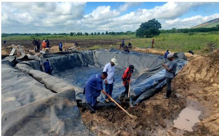
Figure 2: Installation of a dam liner.
