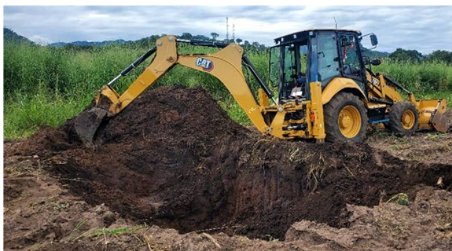
Figure 3: A backhoe is used to dig a retention pond.
